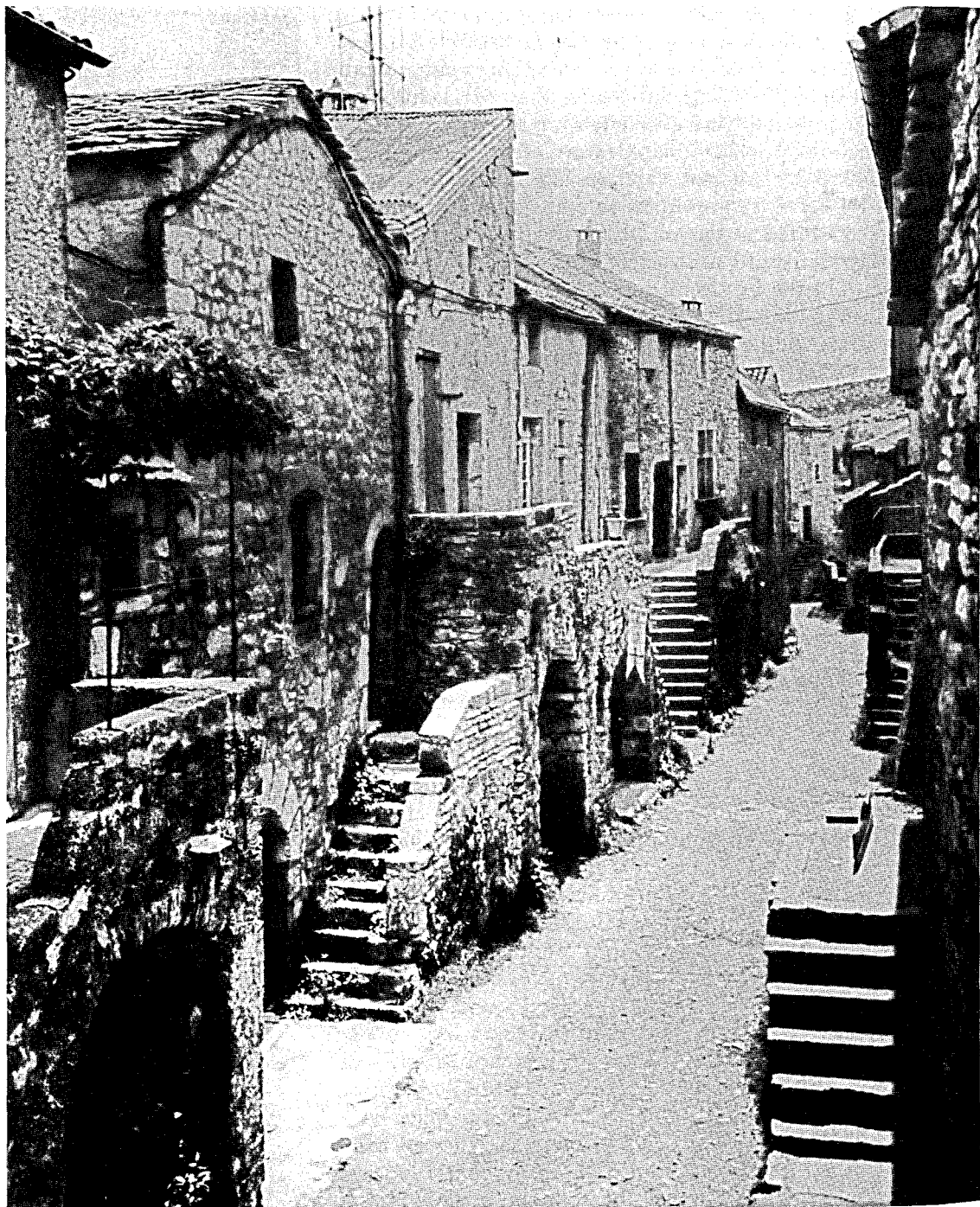
La Couvertoirade (Aveyron). The main street of the village, fortified in the middle of the 15th century on order of its lord, the Order of the Hospital. The stone houses have external staircases that lead to the kitchen and hall; storage rooms are at ground level.
